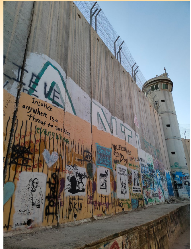
A section of the Israeli separation barrier in Bethlehem, West Bank, Palestine. Photo courtesy of Anthony Khair
