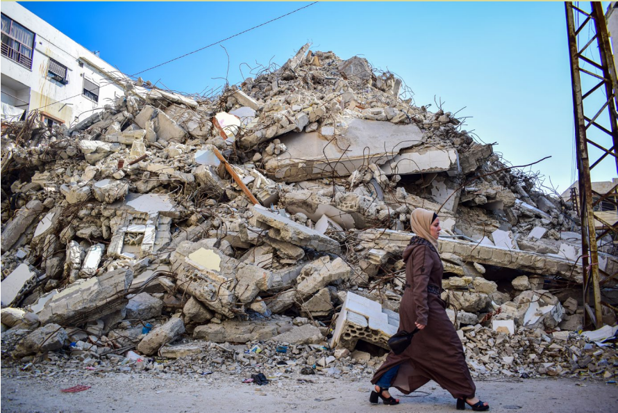
This September 2023 photo shows visible damage from the February 2023 earthquakes is still dominant in the streets of Jabli, a remote city in Lattakia Governorate, Syria. Photo courtesy of Mohammad Said
