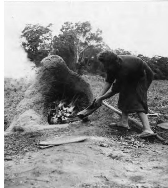
Oven constructed in 1948 in an anthill by Mennonite settlers in the new Volendam colony established by Soviet Mennonites whom MCC helped migrate from Europe to Paraguay. (From Peter Dyck and Elfrieda Klassen Dyck collection, MCC)
